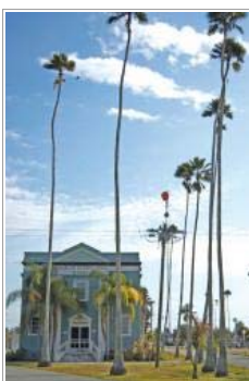
The Bank of Everglades building in Everglades City. COURTESY PHOTO/JANE PIERCE
